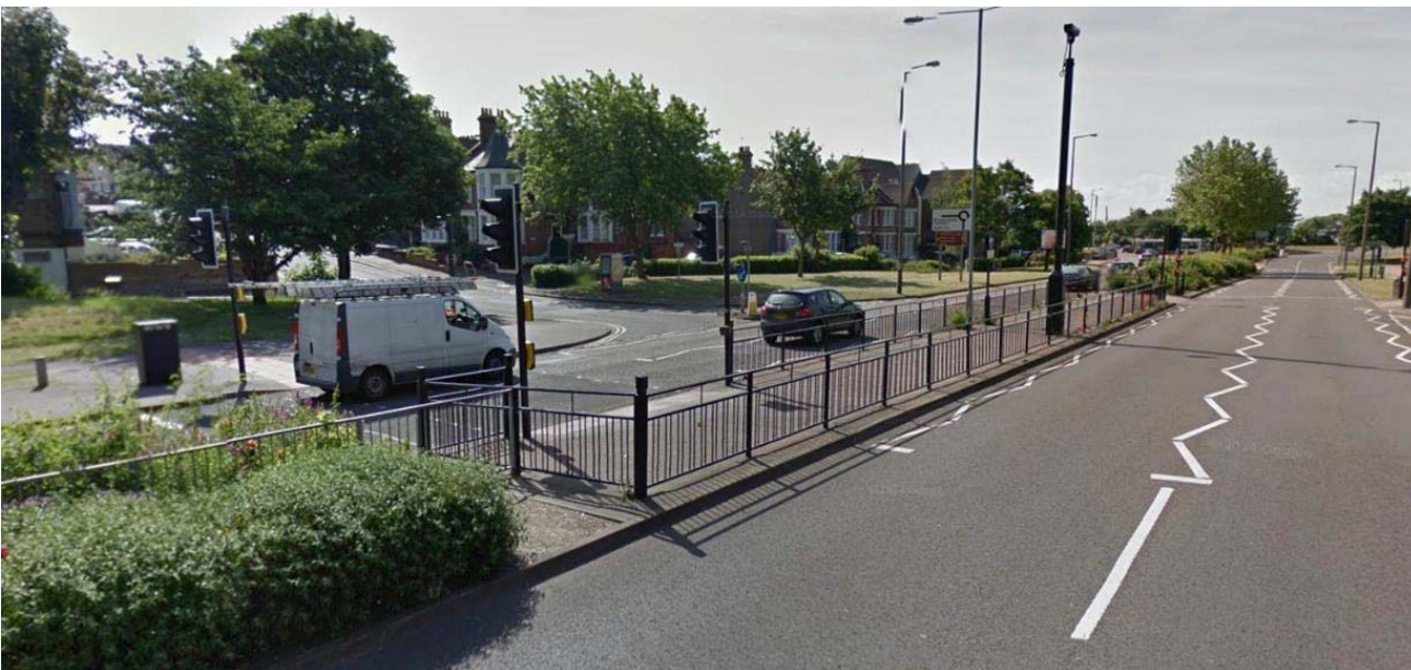
Railings to prevent informal street crossings in the UK
